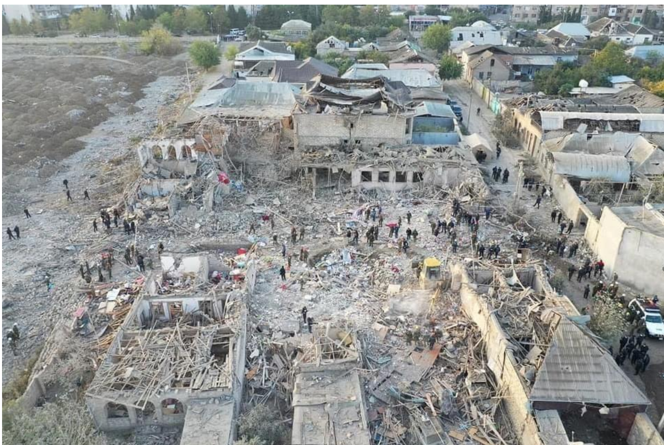
Civilian houses destroyed as a result of the attack of the Armenian Armed Forces on the city of Ganja
